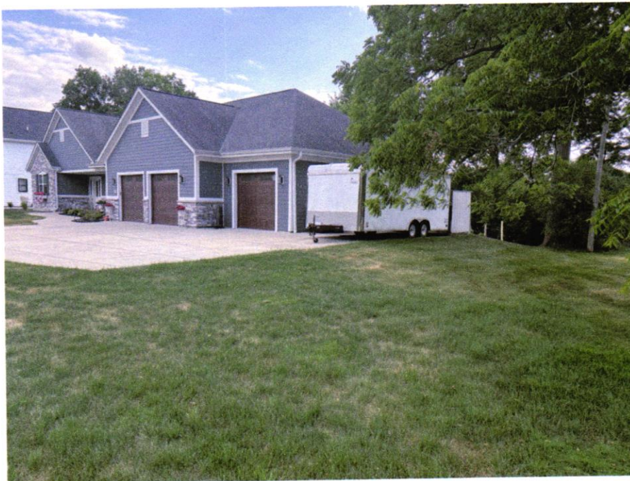
Building location – Looking From Near North Property Line
