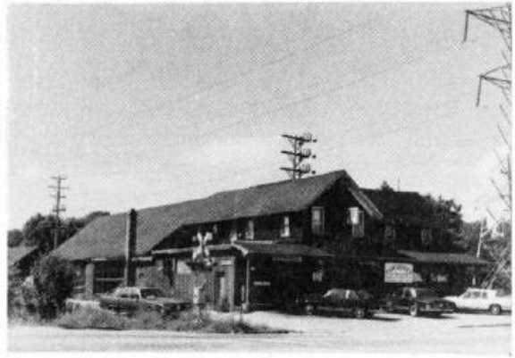
Calhoun Hall in 1988, showing the original wing (r.) the added hotel (l.) and the added dance hall (rear) as well as old outbuildings. The western-style front was added in 1967. Photo by Donald Hermann
