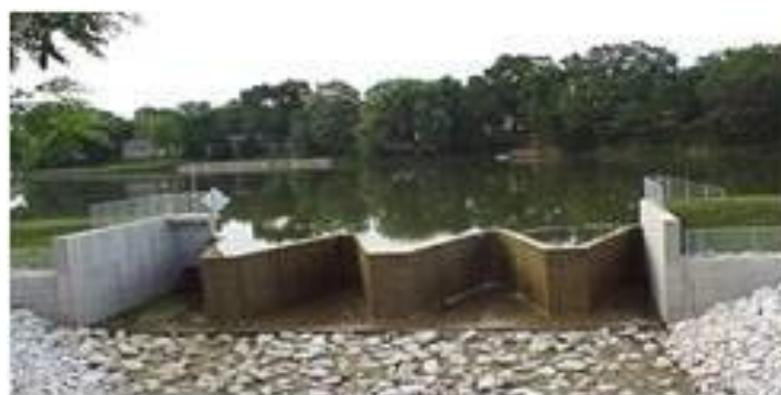
Figure 4.5. Linnie Lac Dam Site
