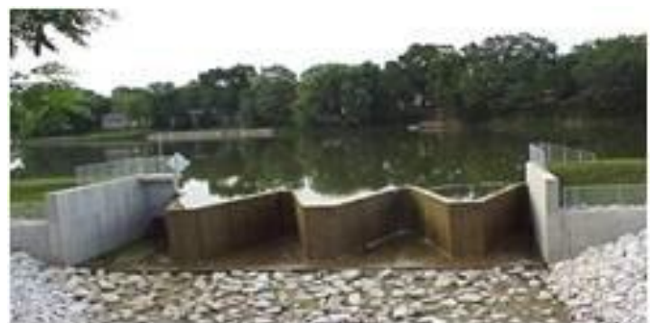
Figure 4.5. Linnie Lac Dam Site
