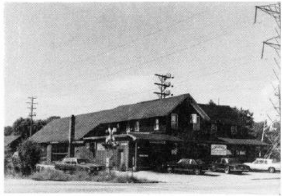
Calhoun Hall in 1988, showing the original wing (r.) the added hotel (l.) and the added dance hall (rear) as well as old outbuildings. The western-style front was added in 1967. Photo by Donald Hermann
