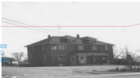
Figure 4.16, Taci's Tavern and Roadhouse
