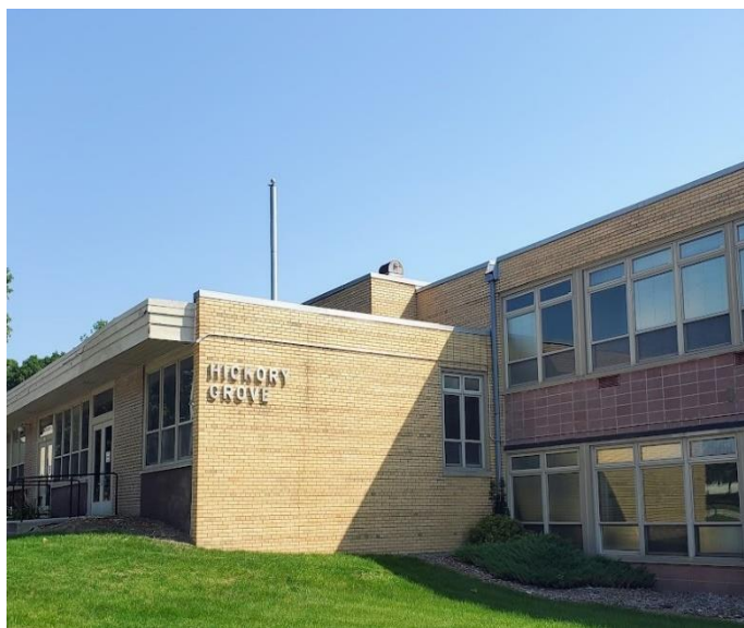
Figure 1: Hickory Grove, 1952 – 2023. Photo taken August 14, 2023
