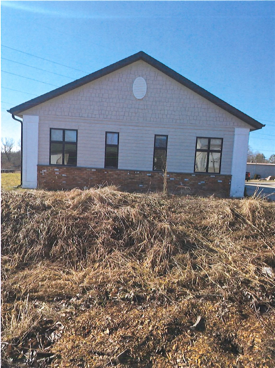
Existing office building
