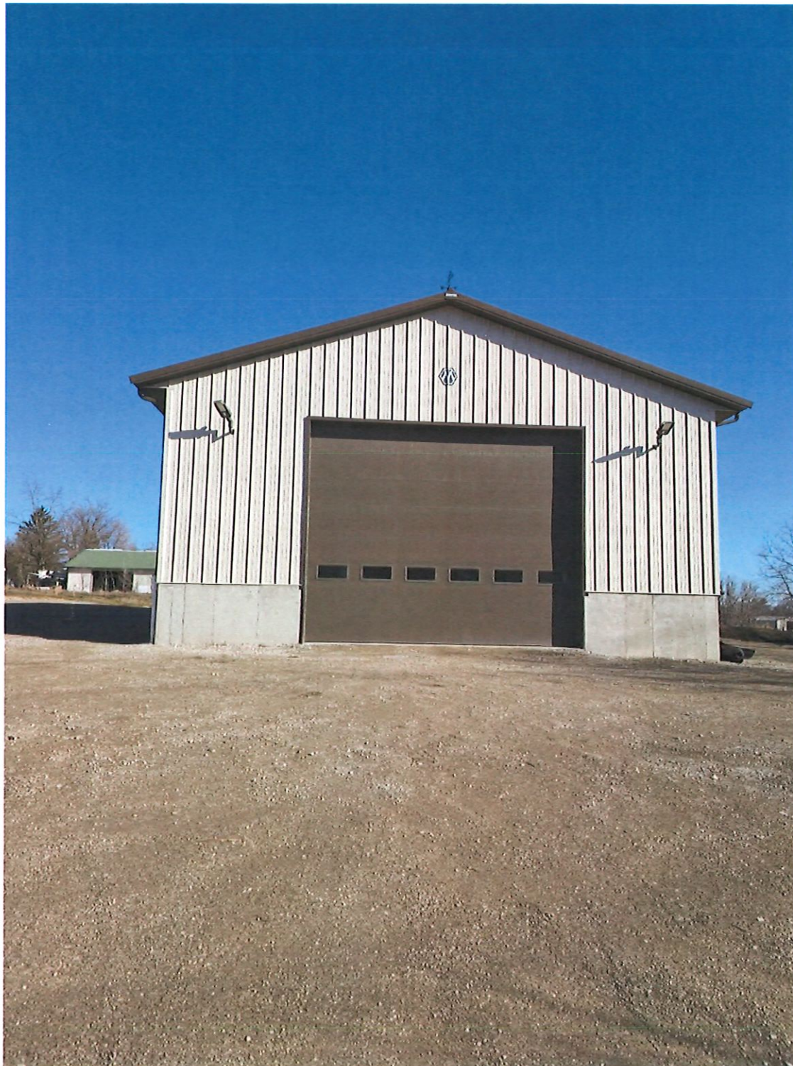
Existing storage building
