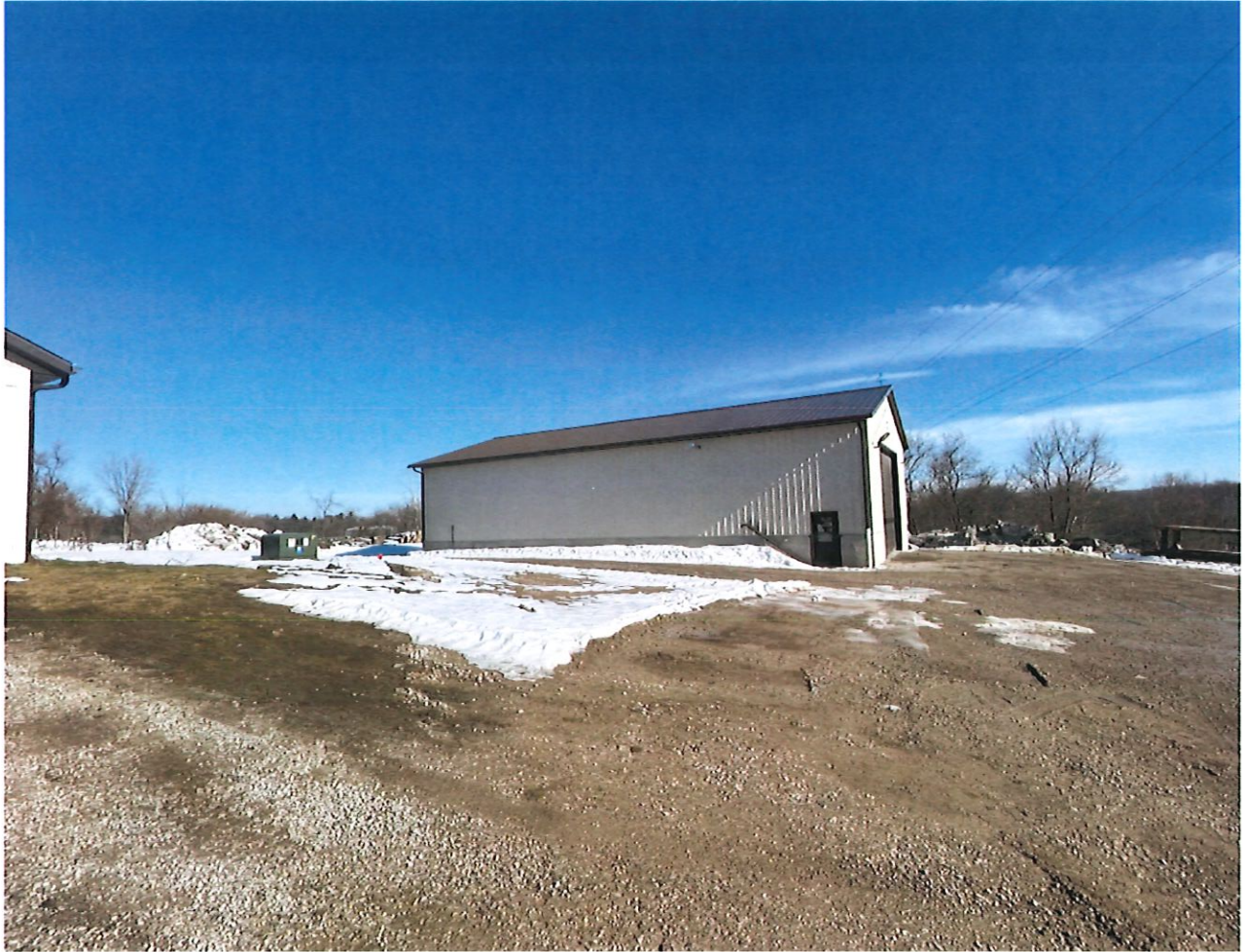
Existing storage building
