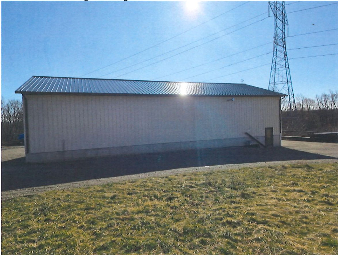
Existing storage building
