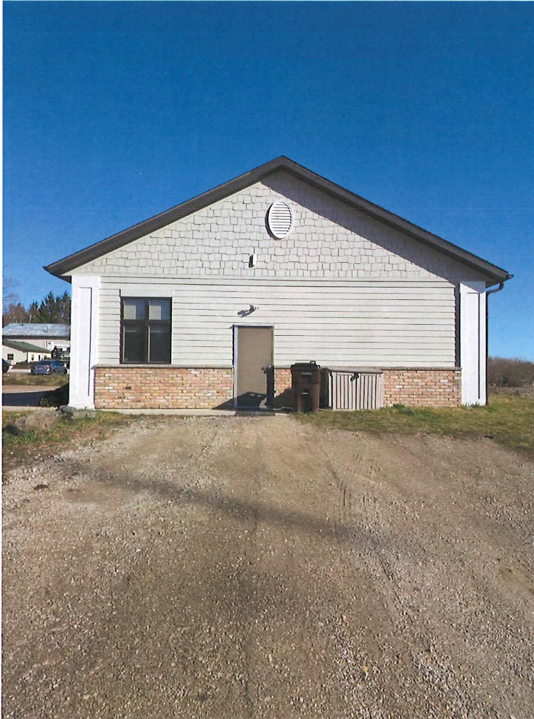
Existing office building
