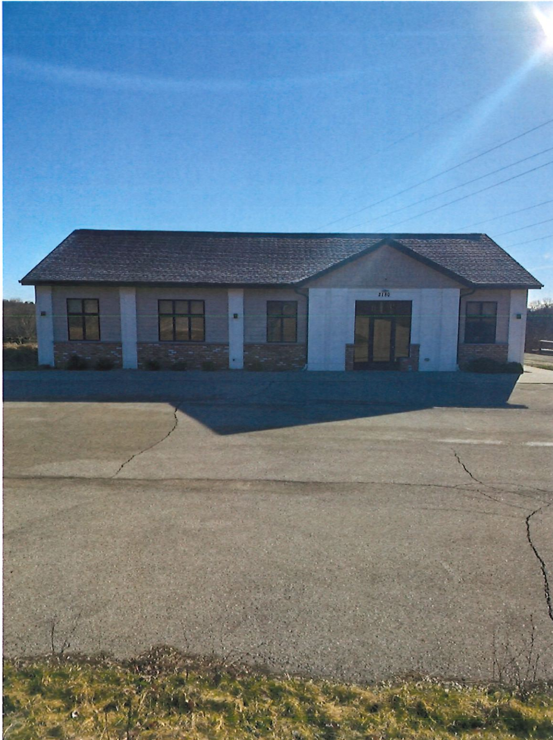
Existing office building
