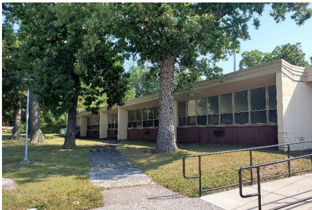
Figure 3: One of additions to Hickory Grove completed in the 1950s. Note the beautiful trees that still surround the school. Photo taken August 14, 2023
