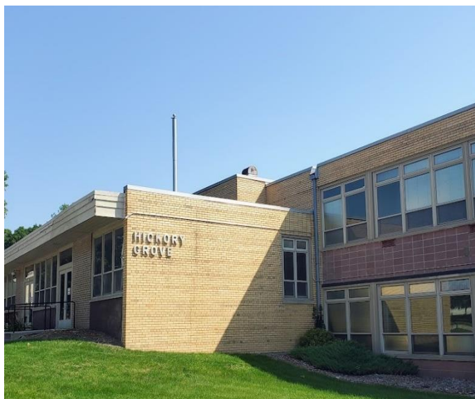
Figure 1: Hickory Grove, 1952 – 2023. Photo taken August 14, 2023
