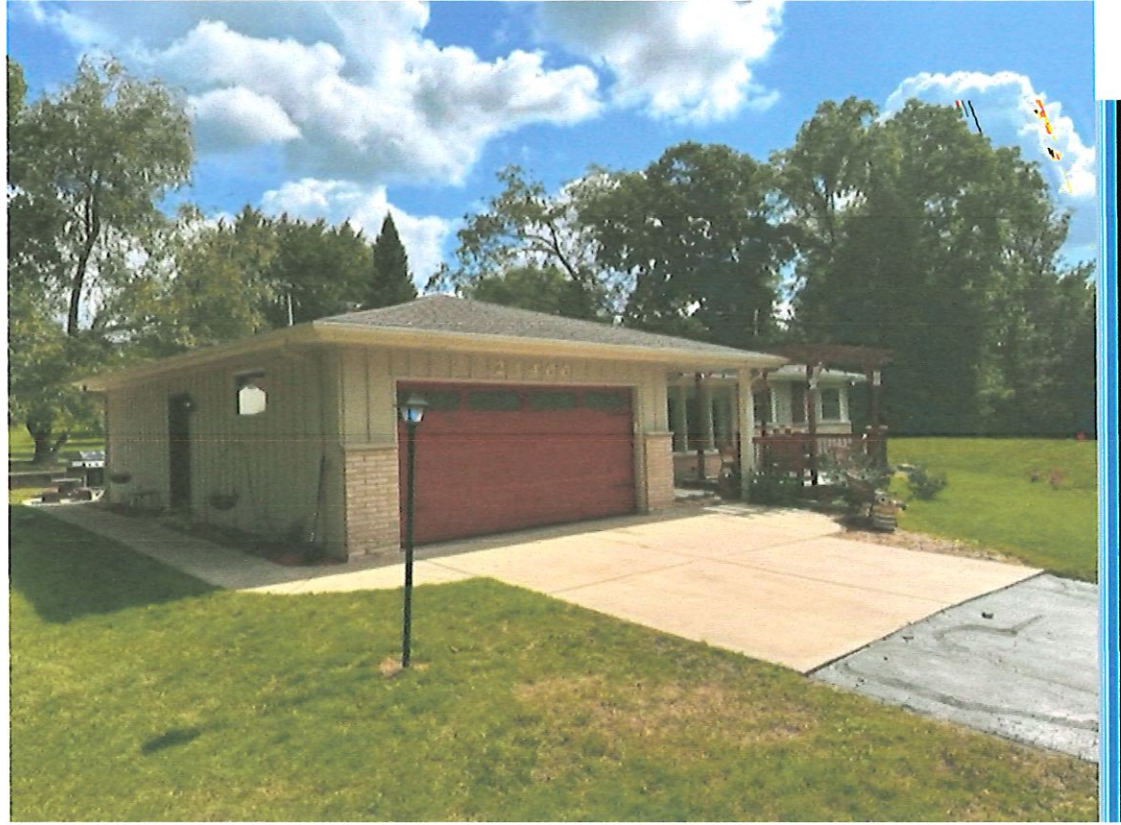
Front and side of house. Notice septic mound in right side of picture.
