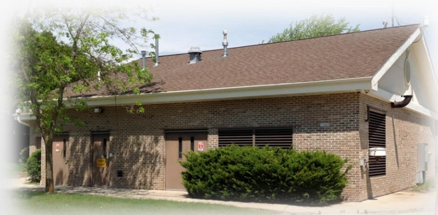
Grange Avenue Pump House Milwaukee #1
