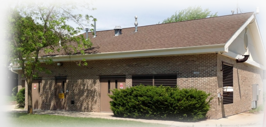
Grange Avenue Pump House Milwaukee #1
