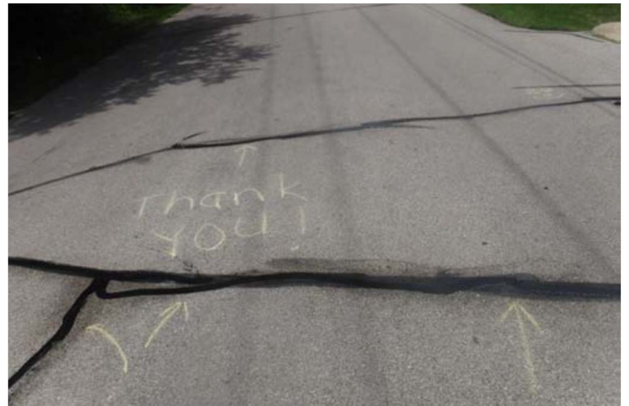
Crack Sealing
