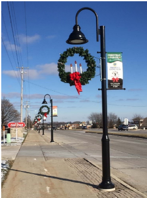
National Ave. Pedestrian Lighting
