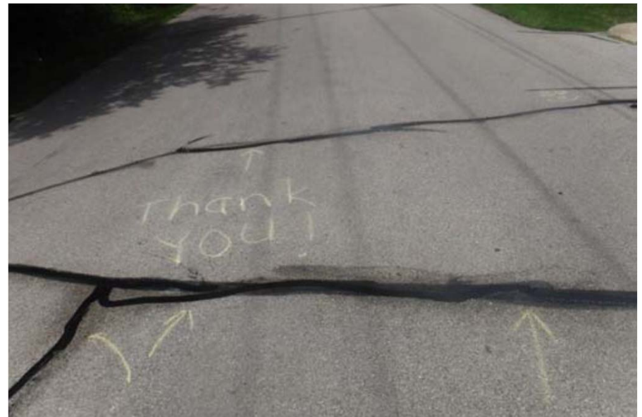
Crack Sealing
