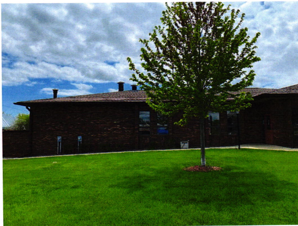
Front Façade – Facing Howard Ave (Location of Proposed Addition)
