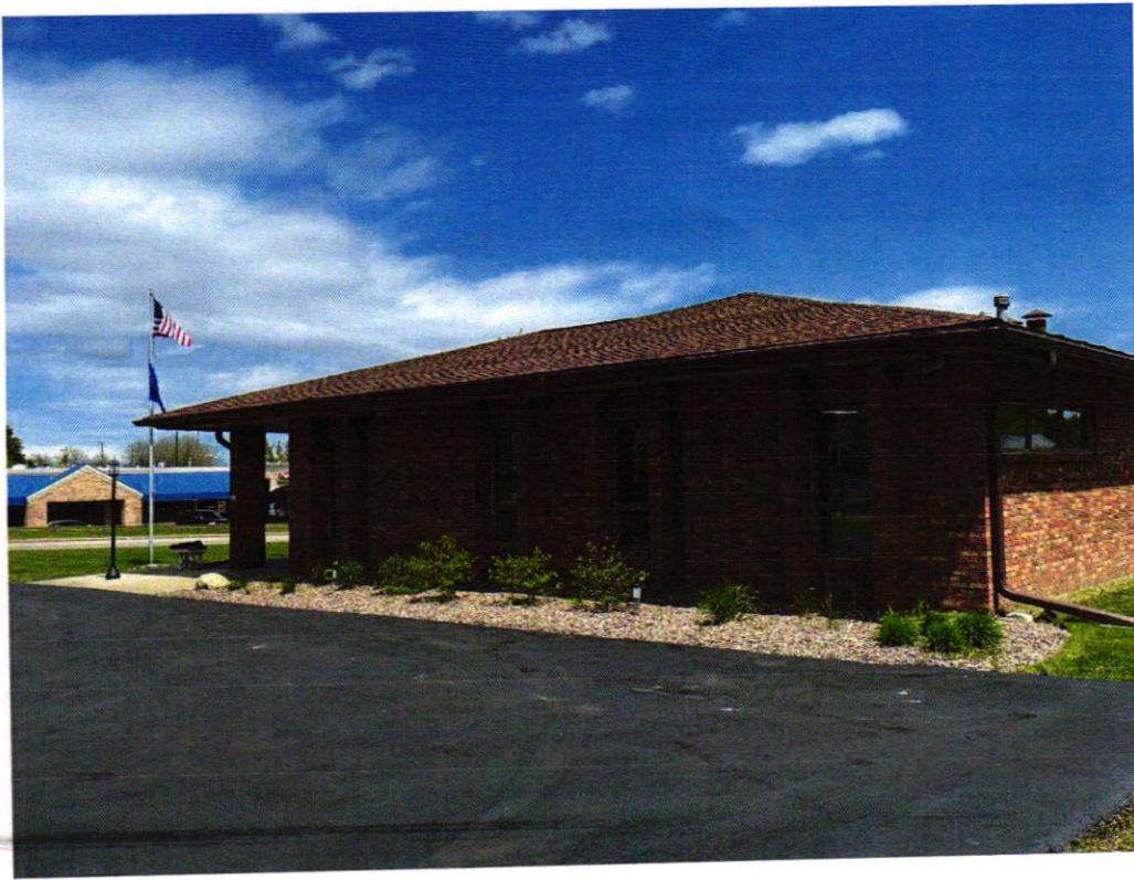
Existing West Elevation – Facing Moorland Rd.
