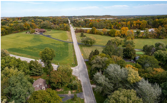
The Small Road project has long-term benefits for the City.
